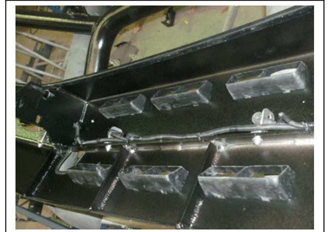
Figure 10: Wiring in rear of Protection Bar
